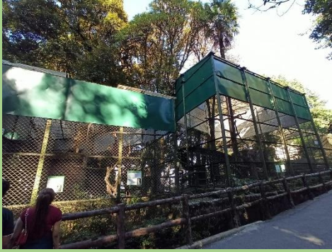
Installation of Visual Barrier at Cockatoo & Macaw Enclosures
