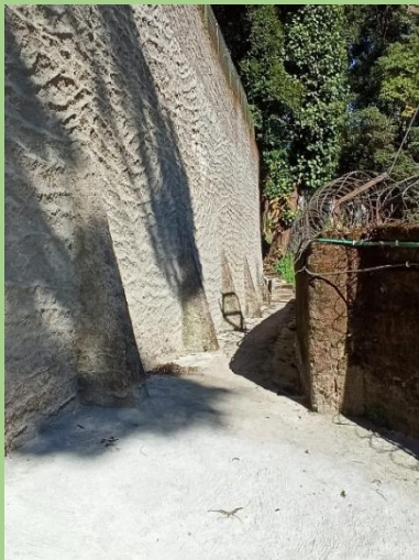
Repair & Maintenance of Service Pathway behind the Herbivore Enclosures 1 – 4
