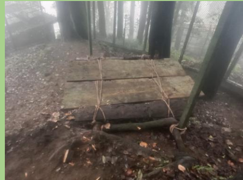
Installation of Wooden Platform at Royal Bengal Tiger Enclosure
